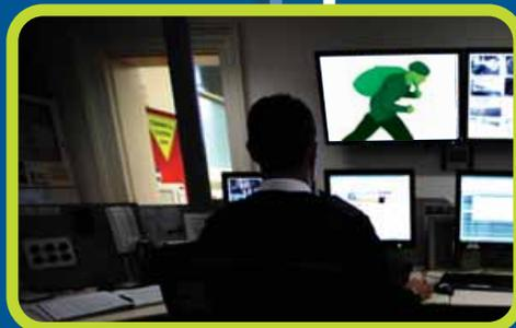
Alarm Notifications are sent to a Central Monitoring Station where an operator sees the video of each alarm and reacts intelligently. Priority Police response is deployed if alarm video is verified.
